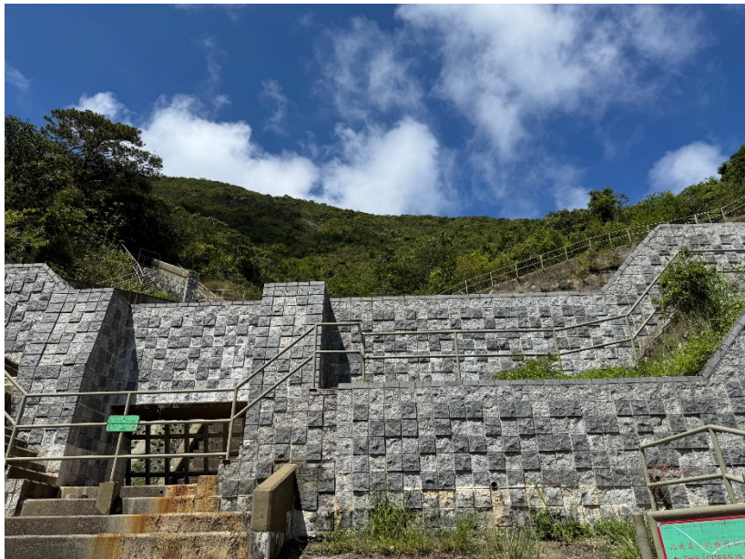
Figure 3: Rigid barrier on Repulse Bay Road (Photo taken by our officer during site inspection in May 2025)
