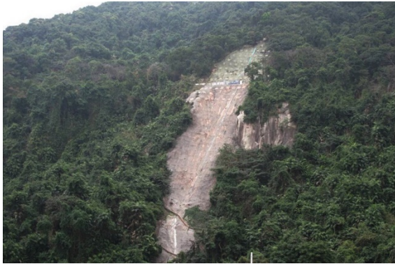
Figure 4: Before upgrading works
