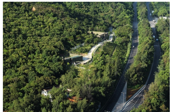
Figure 7: After risk mitigation works
