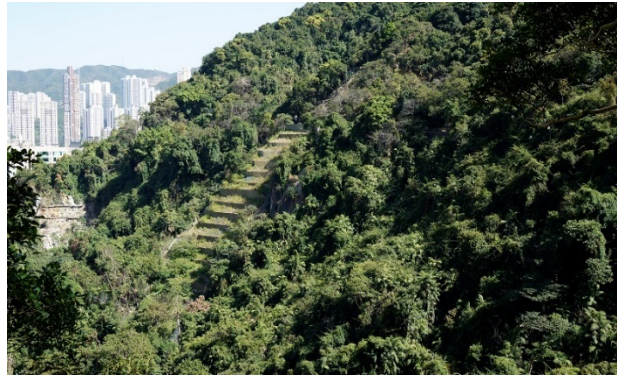
Figure 5: After upgrading works
