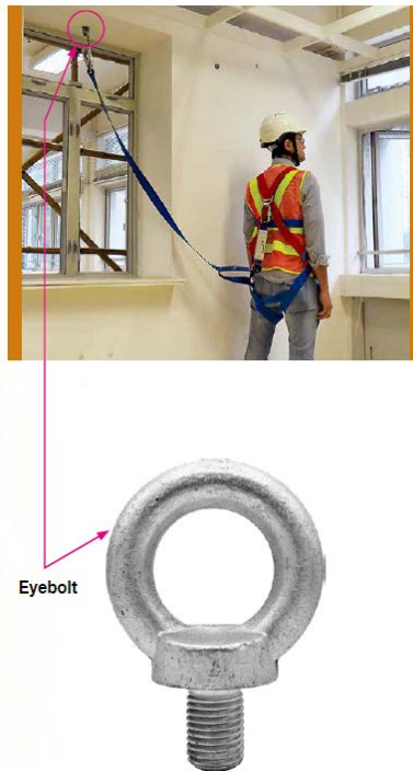
Figure 8: Eye bolt and a worker using an eye bolt (Source: LD's Guide on Construction and Work Safety of Truss-out Bamboo Scaffolds)
