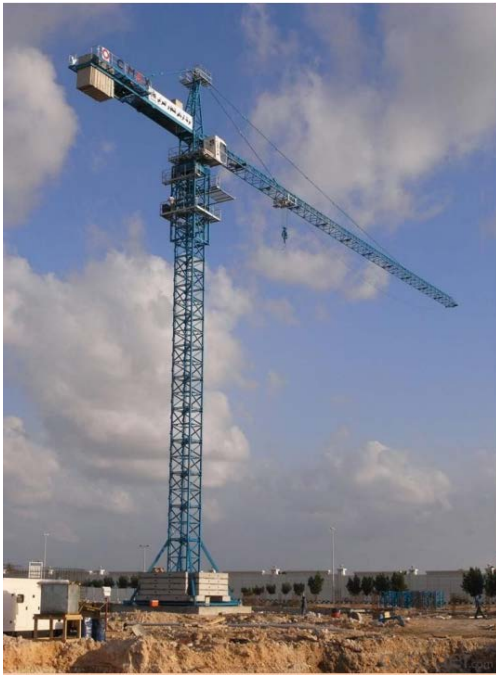
Figure 12: Tower cranes (Source: LD website)
