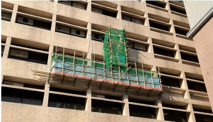
Figure 1: Truss-out bamboo scaffolds (Photograph taken by our staff)
